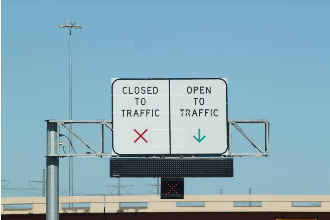
Figure 4. Overhead Static Signing with Lane Control Signal and Single Line DMS.
